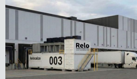
Commercial Facility in Plant City, Florida
