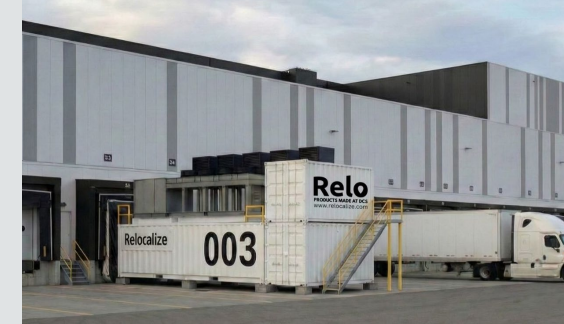
Commercial Facility in Plant City, Florida
