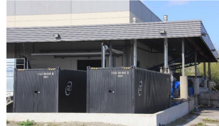
Pilot facility in Delta, British Columbia
